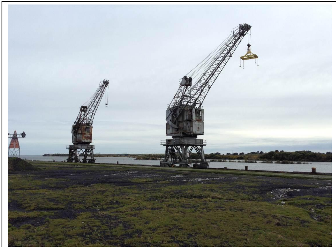
Mike Vincent (Heritage New Zealand), Greymouth Wharf Cranes, 19 September 2013
