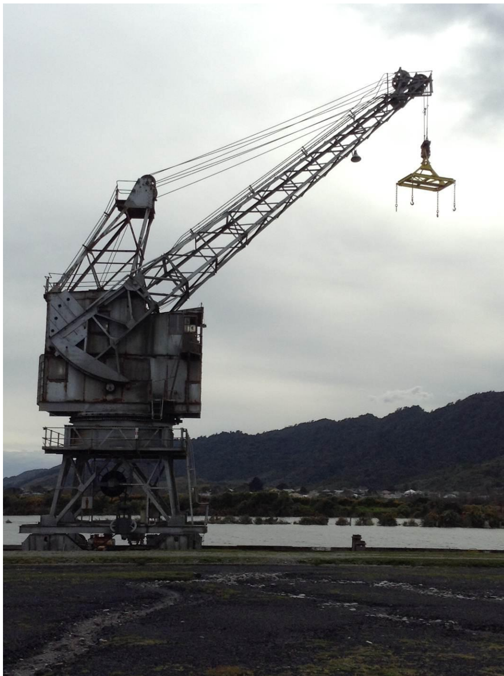
Mike Vincent (Heritage New Zealand, Greymouth Wharf Cranes, 19 September 2013)
