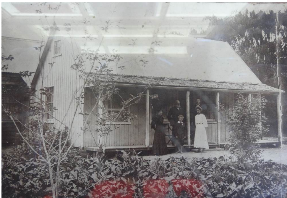
Figure 8: Cottage on its previous site, photograph on display at the Willows Craft Cottage (permission for use granted by Mrs Martini). [This photograph appears to have been taken in the second decade of the twentieth century – it shows the main part of the roof clad in corrugated iron, whereas the photo dated 1911 shown at Figure 7 above shows the whole of the roof was shingled. Note a building to the rear].
