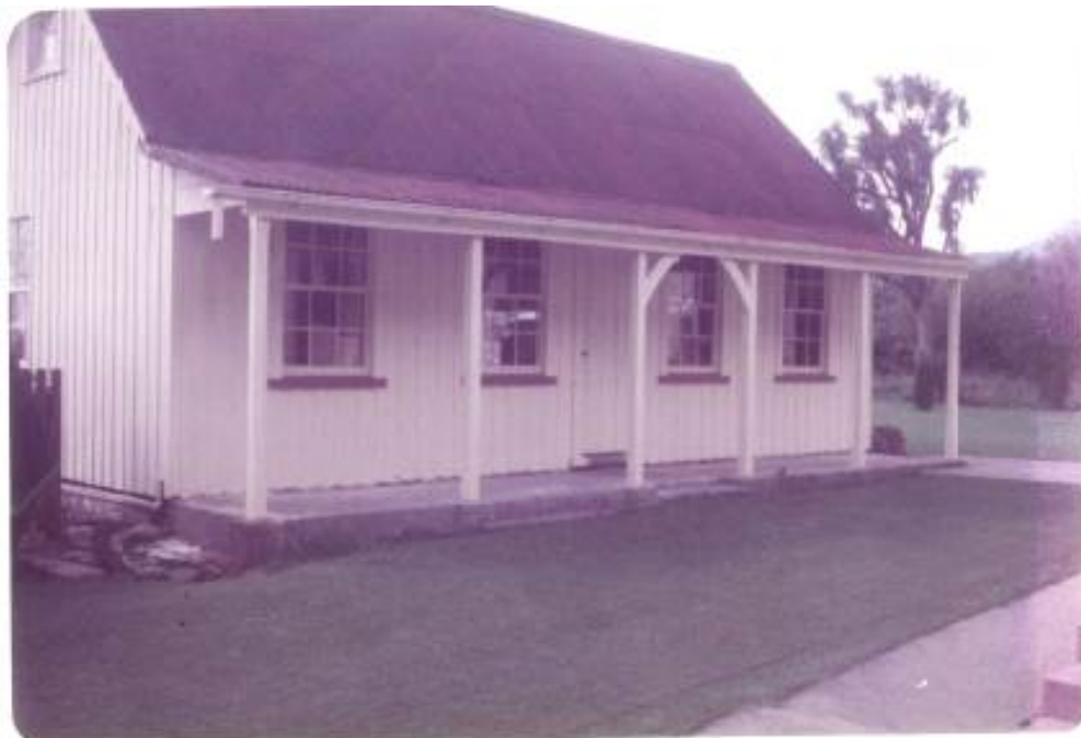
Figure 10: 'Jim Hende Home, Hari Hari', Molly Martini, 1980s, [this is the cottage on its original site, before relocation].
