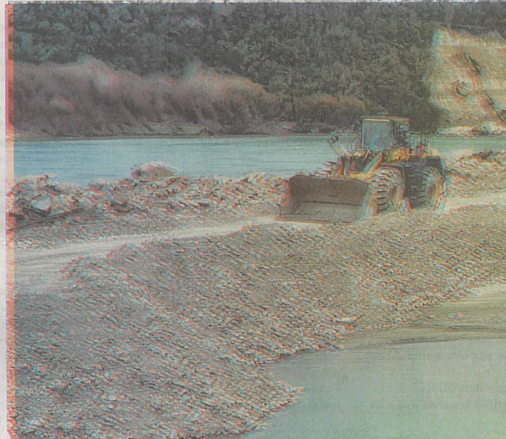
Avery Bros rebuilding the Organs Island rockwall in August, 2022. Photo: Flag M
