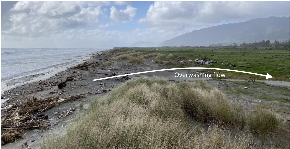
Figure 4-4: Wave overwashing through dune erosion and blowouts at Collins Rd. Overwashing deposits (sands and gravels) deposited 30 m inland from beach face. Date: 13.8.2021 [Credit: M. Allis (NIWA)].
