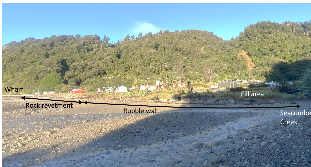
Figure 4-42: Jackson Bay village coastline with new rock revetment at the terminus of the Wharf transitioning to rubble wall wrapping around to Seacombe Creek. Note low-lying fill area/carpark adjacent to Creek mouth. Date 12.8.2021 [Credit: M Allis (NIWA)].
