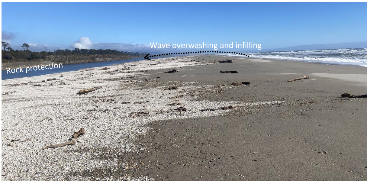
Figure 4-32: Recent rock protection for Haast-Jackson Bay Road alongside cutoff lagoon branch north of Okuru River (at left) with evidence of recent wave washover deposits in filling the lagoon branch (foreground). Date 12.08.2021 [Credit: M Allis (NIWA)].
