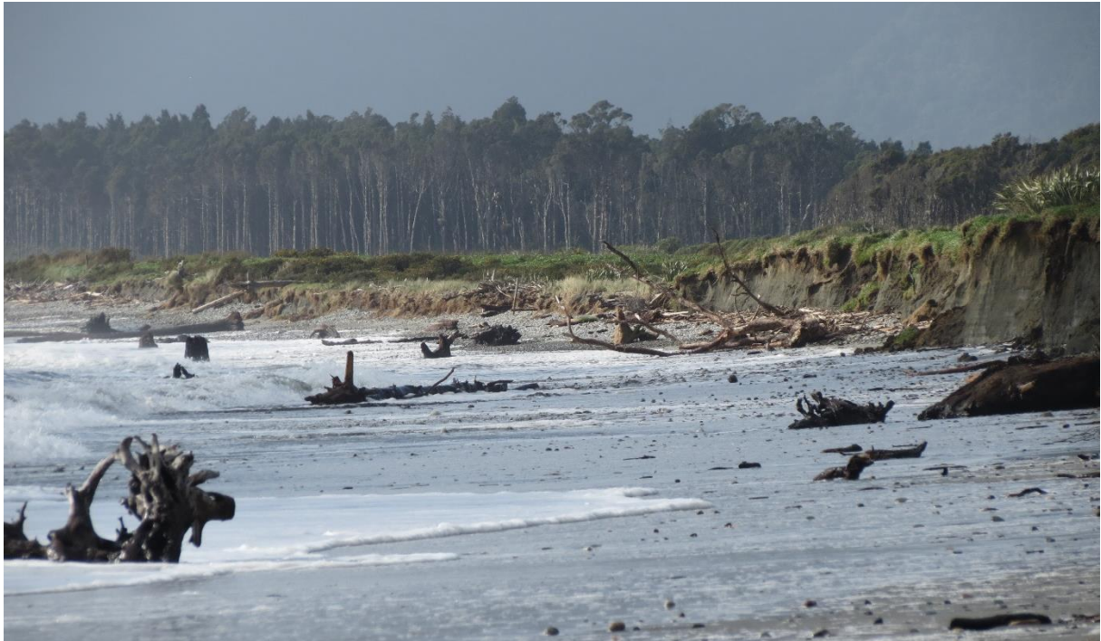
Figure 4-3: Erosion with 2-3 m scarp to the north of Beach Road towards the Whareatea River in CHA3 . Tall trees in distance are located on the north bank of the Whareatea River mouth. Date: 13.8.2021 [Credit: M. Allis (NIWA)].
