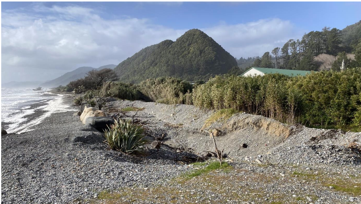
Figure 4-6: Erosion north of Gravity School revetment with drain infilled, berm eroded and vegetation rolling back towards private property. Date: 13.8.2021 [Credit: M Allis (NIWA)].
