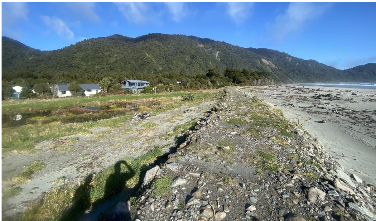
Figure 4-37: Neils Beach village with sacrificial bund (foreground) separating the active beach face from the lagoon and low-lying inhabited land. Date 12/8/2021. [Credit. M Allis (NIWA)].
