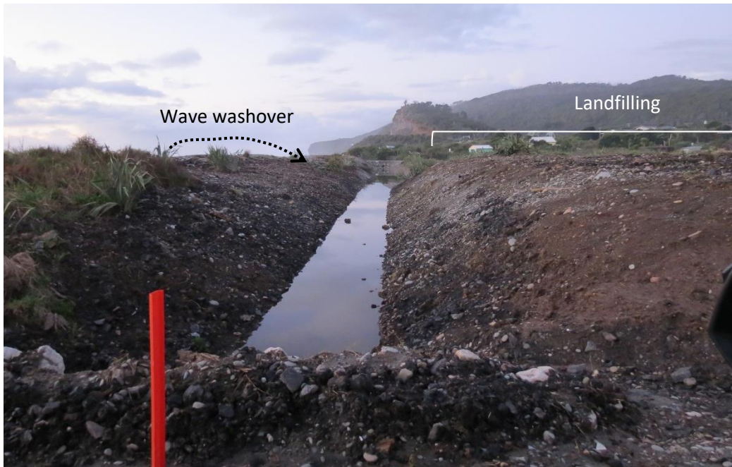
Figure 4-26: Rapahoe drain aimed at capturing wave overwash while infilling of the hindland was used to reduce inundation hazard (right).
