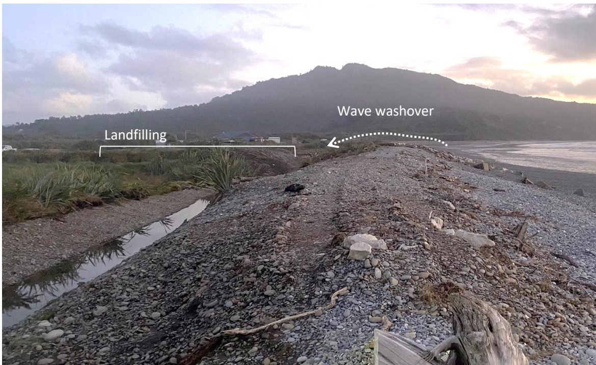
Figure 4-24: Aftermath of wave overwashing at Rapahoe following exTC Fehi. Note driftwood debris spread up to 50 m inland from the beach face, washover of gravel enveloping Beach road and spreading into flax bushes and flooding inundation of low-lying areas and blocking of drains. Also note the scattered rock from the damaged revetment. Note section with busses since infilled to increase land elevation. [Credit: WCRC].
