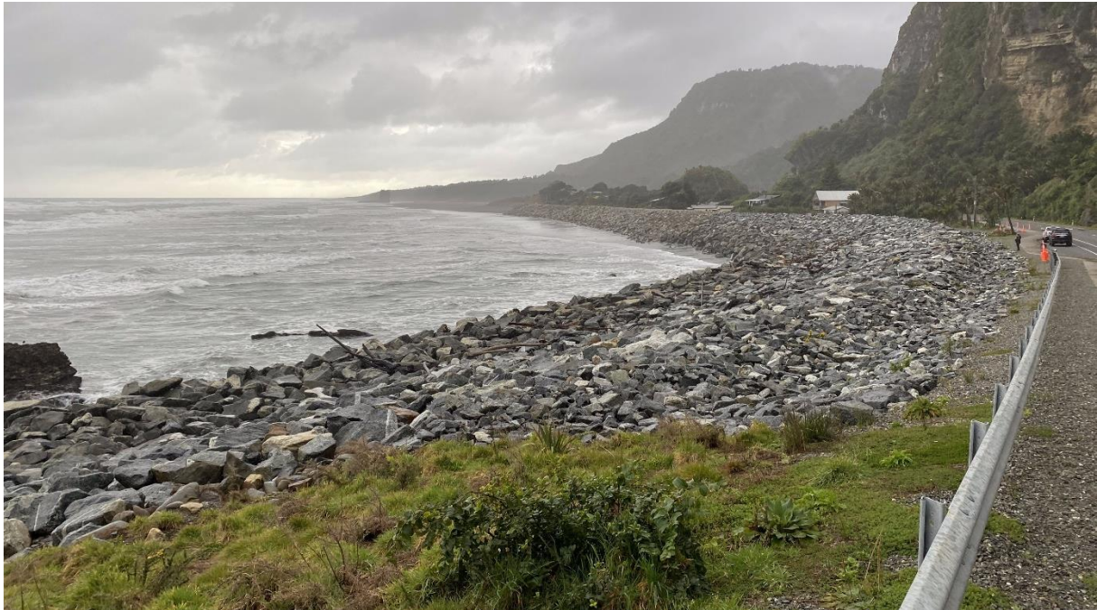
Figure 4-16: Punakaiki Village with coastal protection structures. Date 13/8/2021. [Credit: M Allis (NIWA)].
