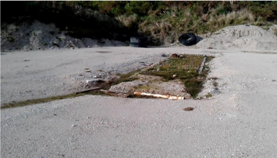
Photograph 3: Former AST footprint.
