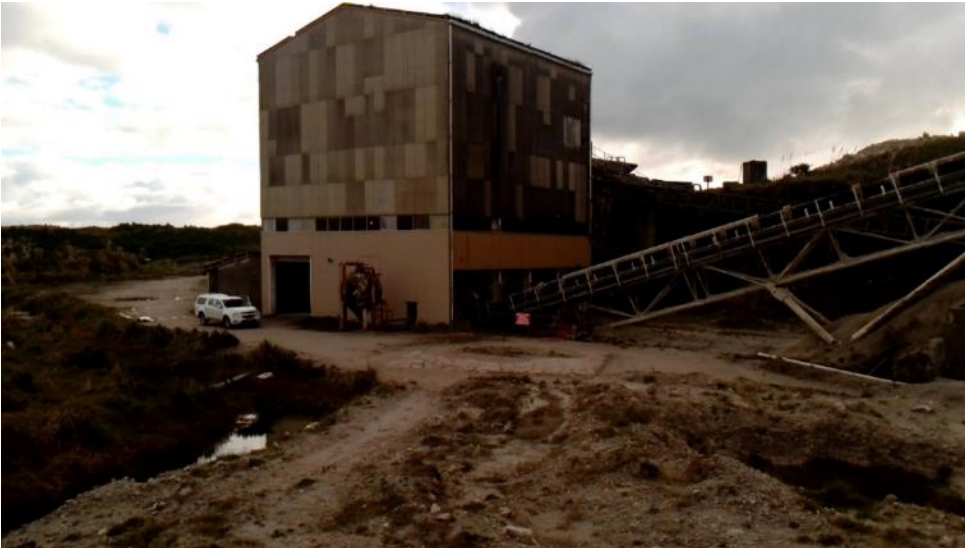
Photograph 20: Crusher – facing north.
