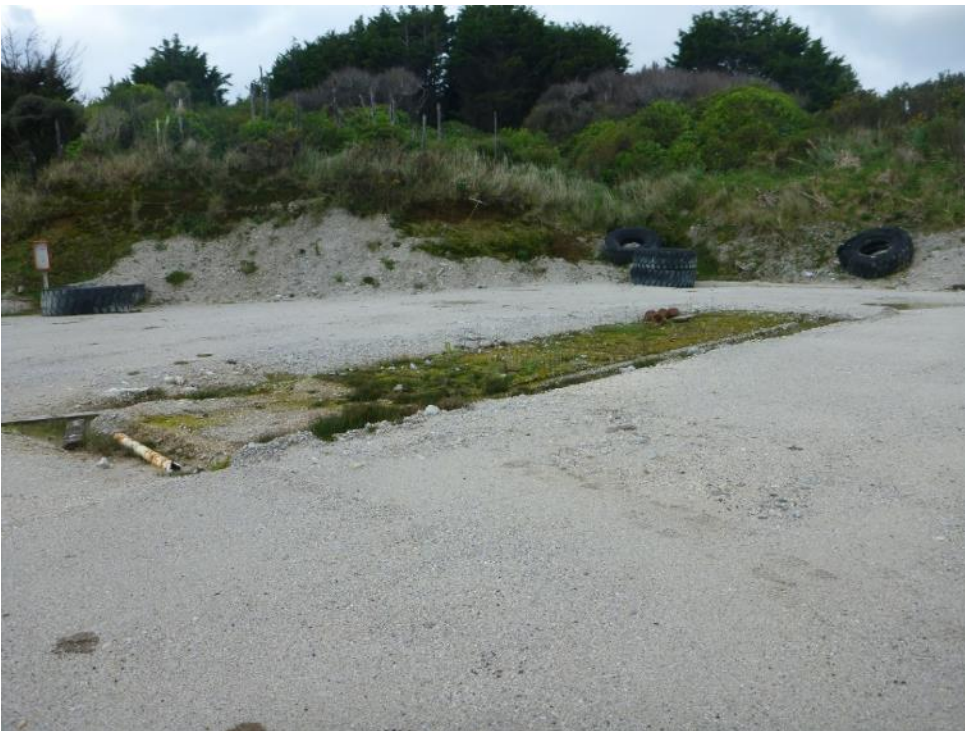
Photograph 4: Former AST footprint.
