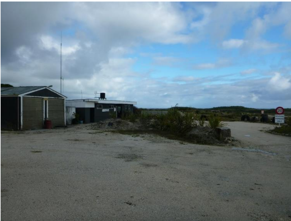
Photograph 2: Main entrance – facing south.
