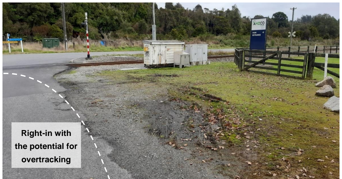
Figure 1: Grassed shoulder on Blair Road near the intersection of Arnold Valley Road showing several tyre tracks from vehicles manoeuvring and/or parking on the shoulder. Photo taken on 17 May 2024.
