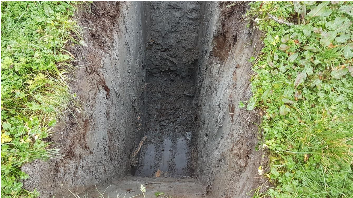
Figure 6. Photo of test pit 09
