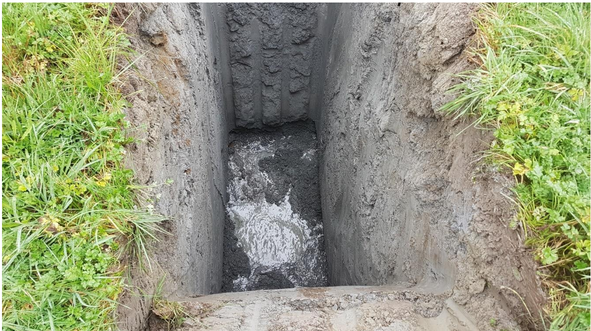
Figure 4. Photo of test pit 06
