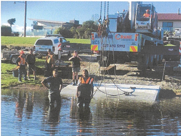
100 tonne crane required to lift panels into place.
