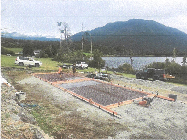
Boat ramp pad construction , 13 tonnes each.
