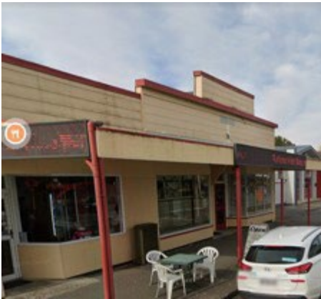
Roofline hidden behind parapet
