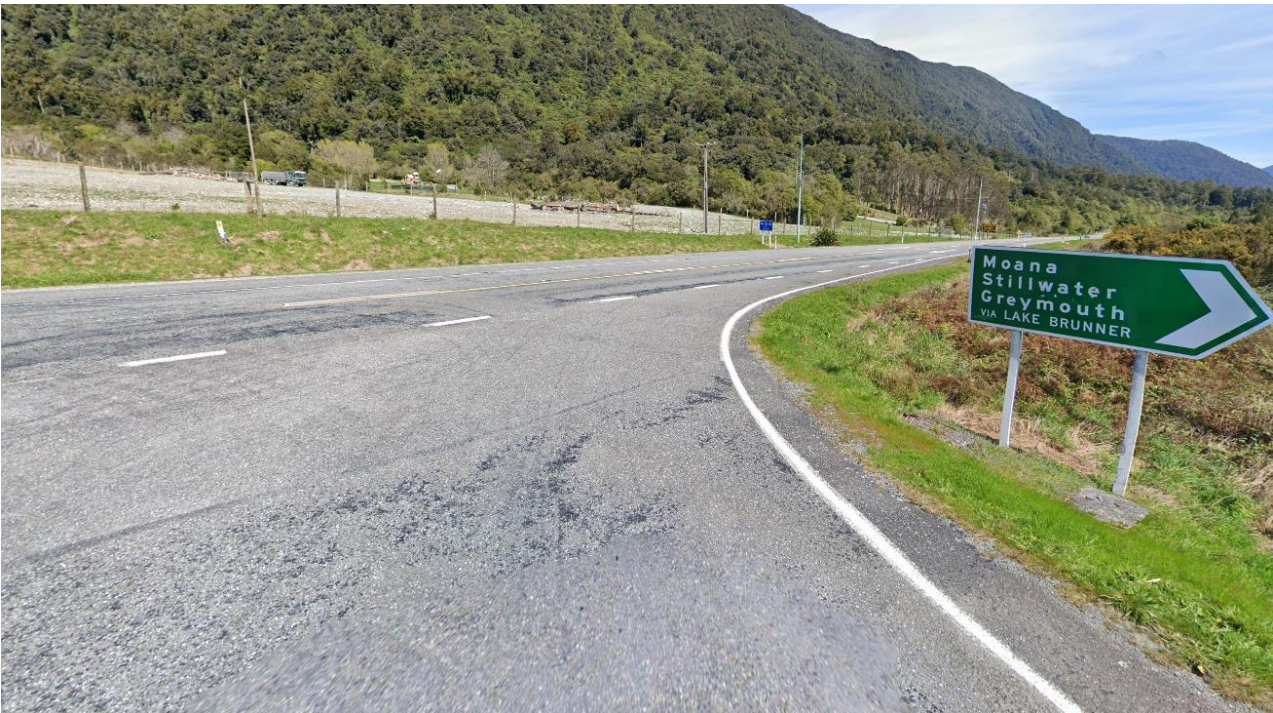
Figure 8 Looking right (west) on Lake Bruner Road to SH73
