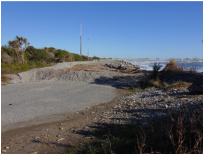
Photo 2 Domett Esplanade, Cobden. Extension pre the high spring tides of Thursday 1 August 2019. Note the wave deposited Grey River flood driftwood. Photo author
