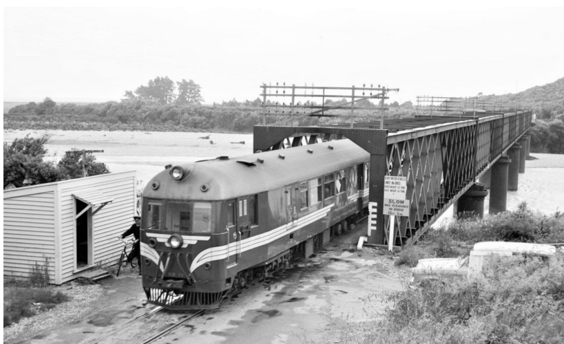
The bridge in 1964. West Coast Recollect.
