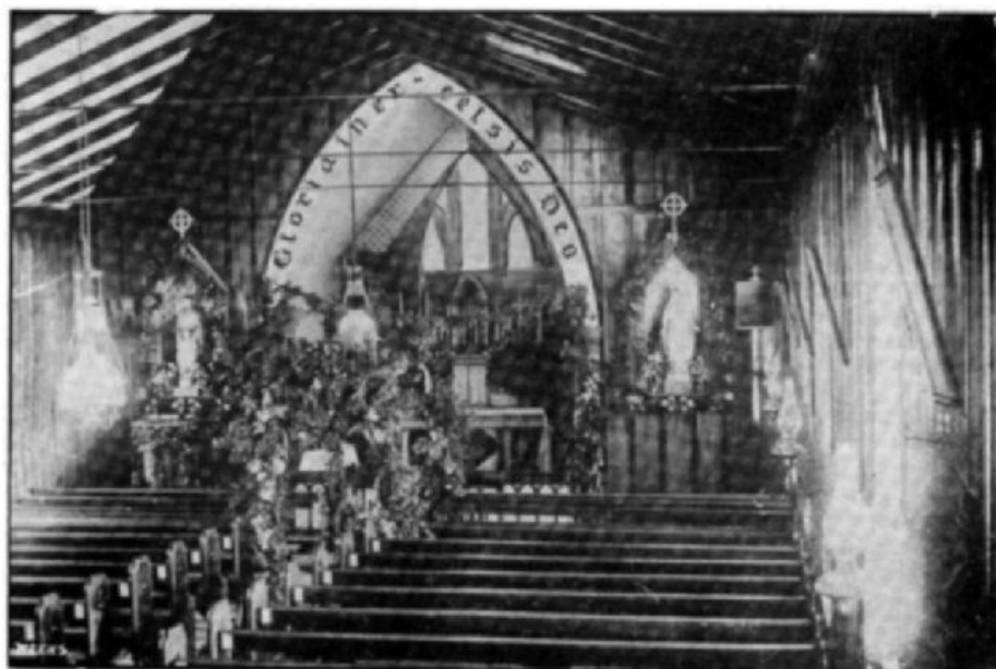
INTERIOR OF ST. PATRICK'S CHURCH, KUMARA.
