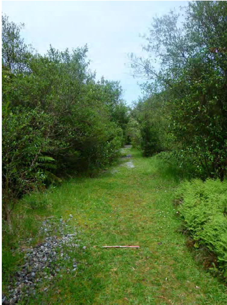
Figure 10. Looking west along the Chasm Stream railway line, waypoint 736. Ballast is visible on the embankment.
