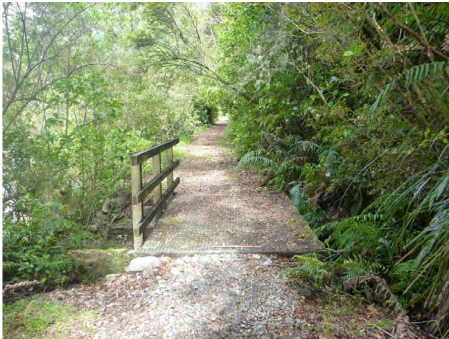
Figure 18. Footbridge 2 at waypoint 745, looking east.
