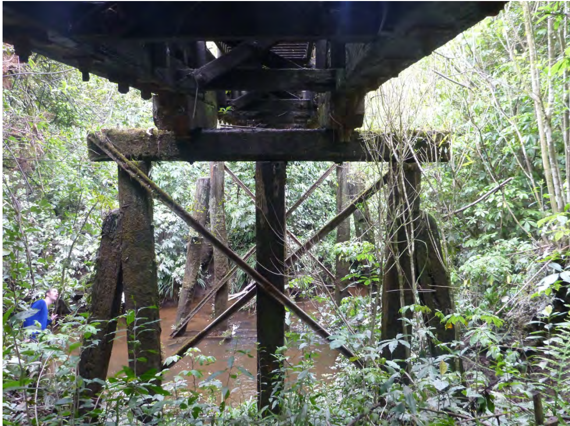
Figure 32. Looking east under Bridge 37, with Pier 2 in the foreground.
