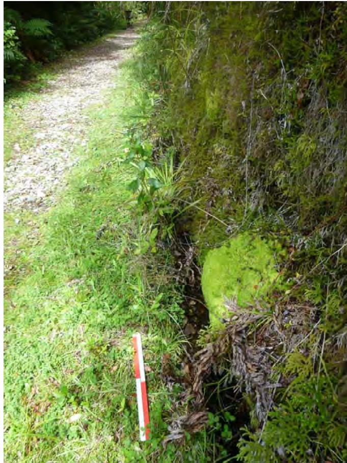
Figure 13. The side drain in the cutting in Figure 11.
