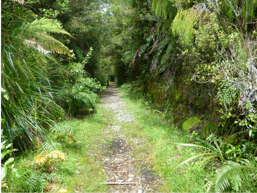
Figure 11. Looking east down the cutting at waypoint 744. This is 3.6 m wide at the base and approximately 27 m long, with a side drain on the south (right) side.
