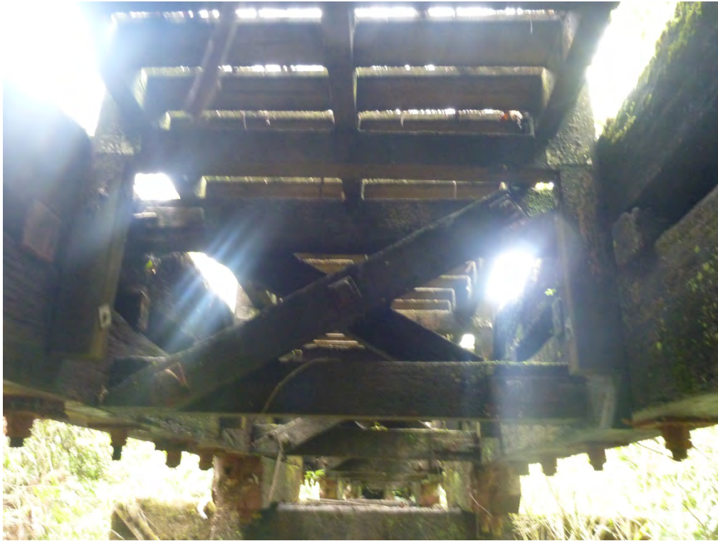
Figure 30. Cross-bracing under the bridge decking, Bridge 38.
