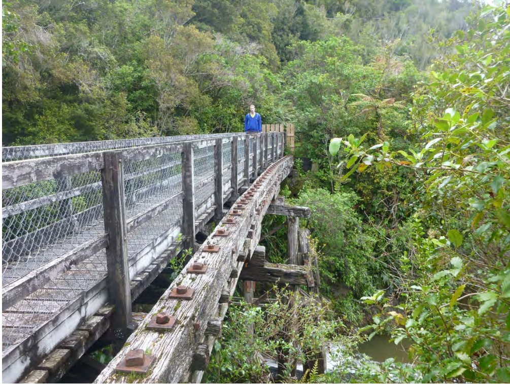
Figure 23. Looking west along Bridge 23.
