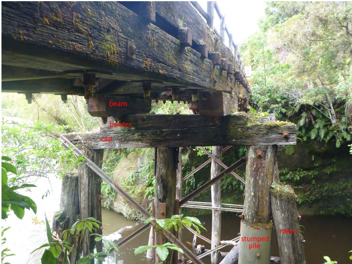
Figure 27. Pier 2, with various components labelled.
