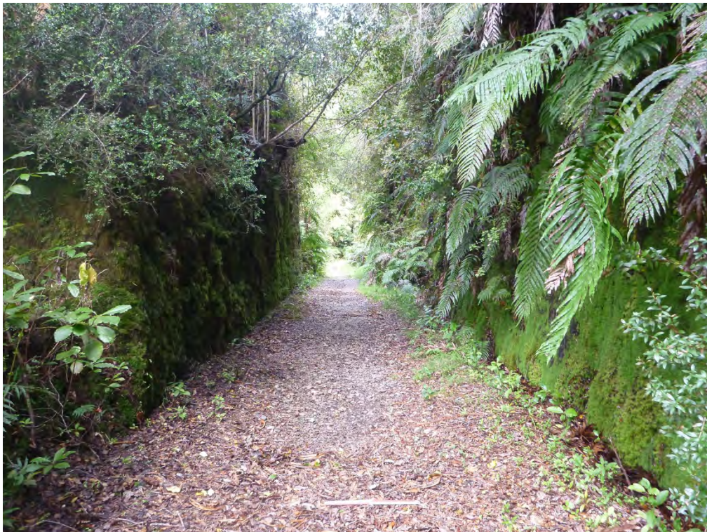
Figure 12. The cutting at waypoint 746. This was 23 m long, and 3.7 m wide, with a side drain on the south (right) side.
