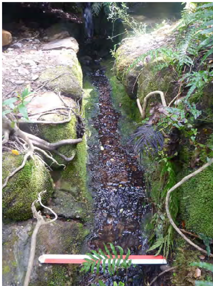
Figure 19. The stone-lined channel under Footbridge 2.
