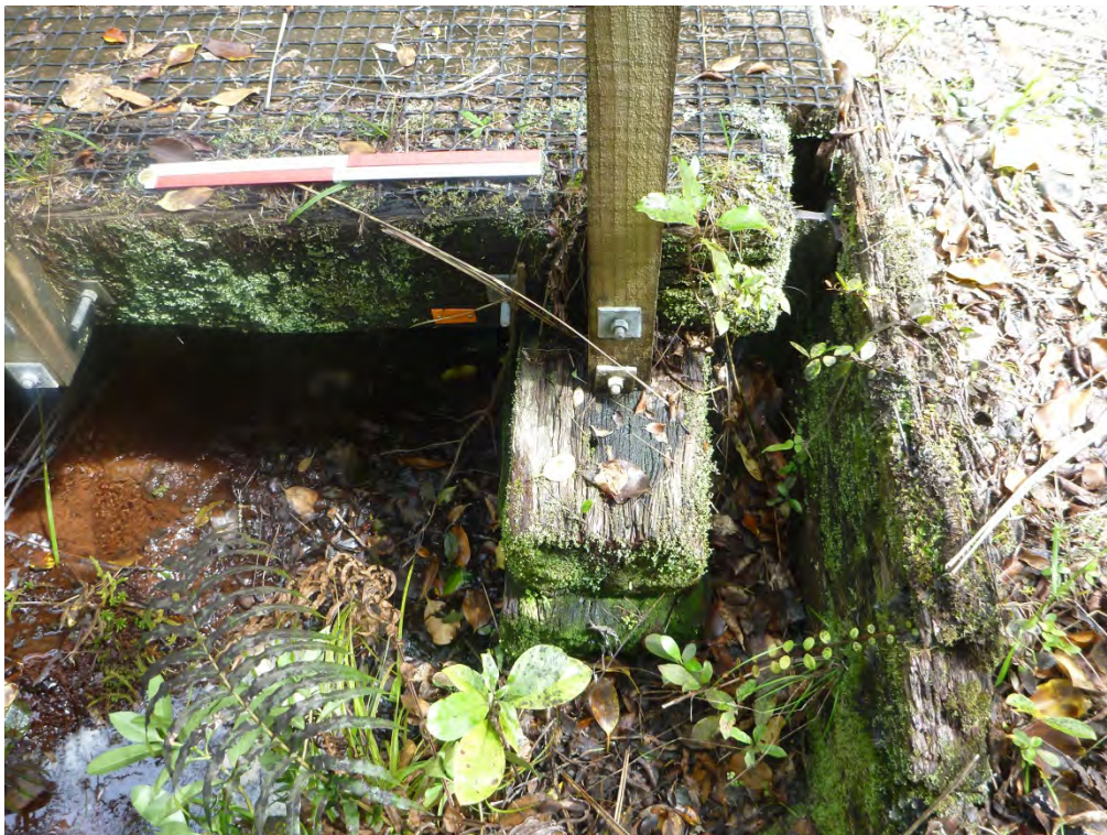
Figure 17. The west end of Footbridge 1, showing the ballast guard at that end.
