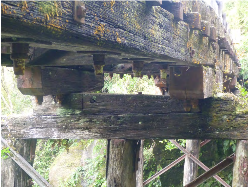
Figure 25. The structure of the spans, Bridge 37.
