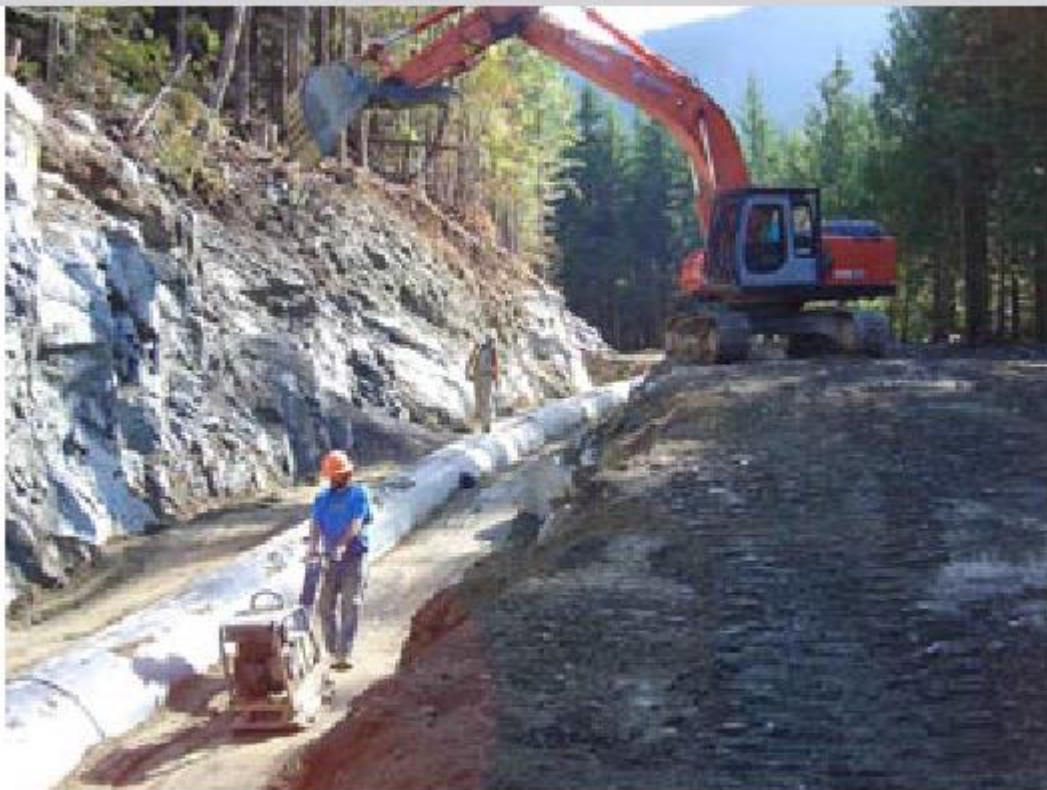
Construction of the penstock at Furry Creek. IPPBC photo.
