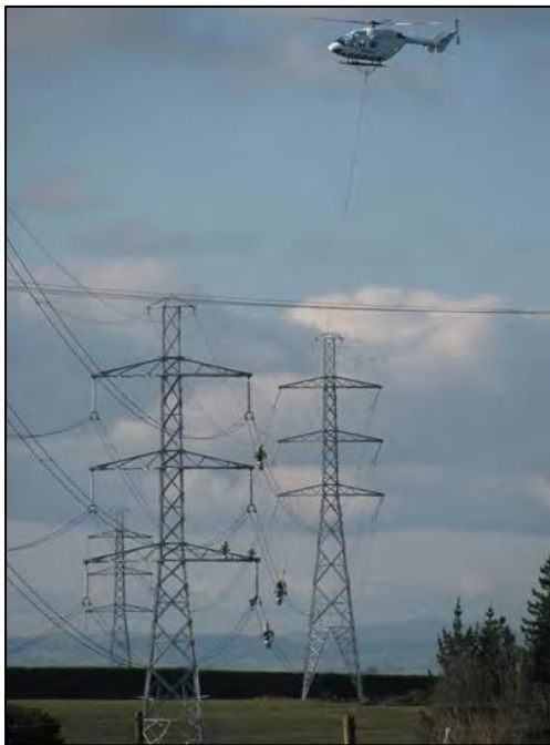
Figure 13 Maintenance work being carried out using helicopters.
