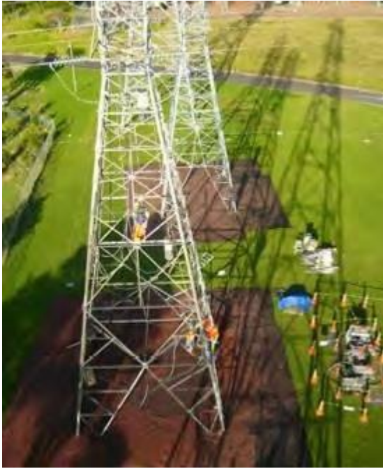
Figure 12 Abrasive blasting in area with no under-build.
