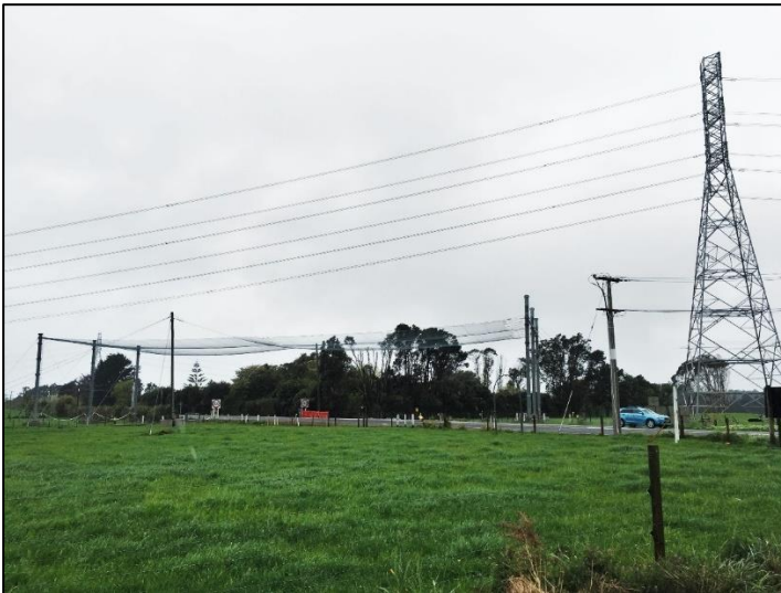
Figure 18: More substantial hurdles installed to mitigate potential conductor drop during wiring.
