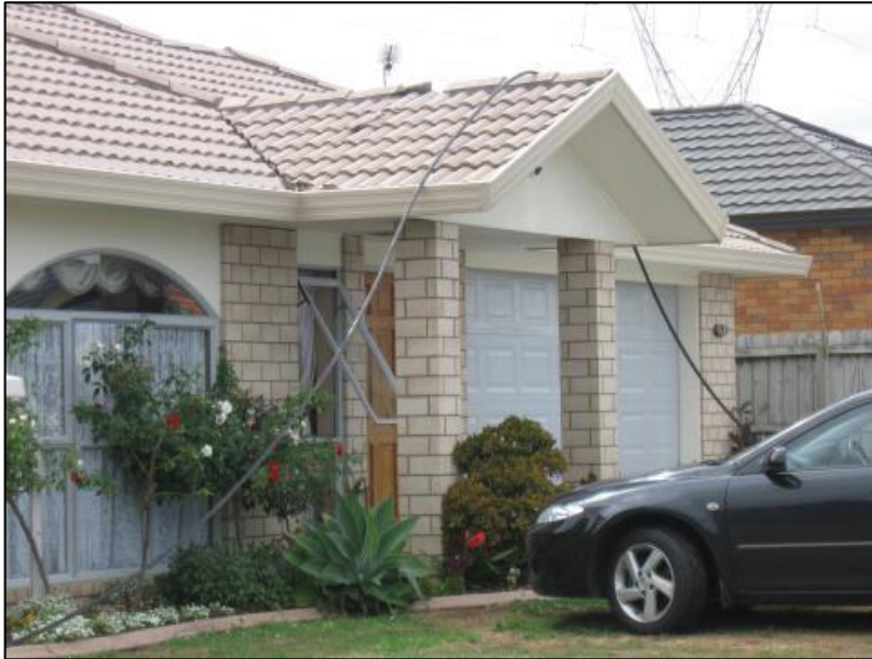
Figure 2 Conductor drop.
