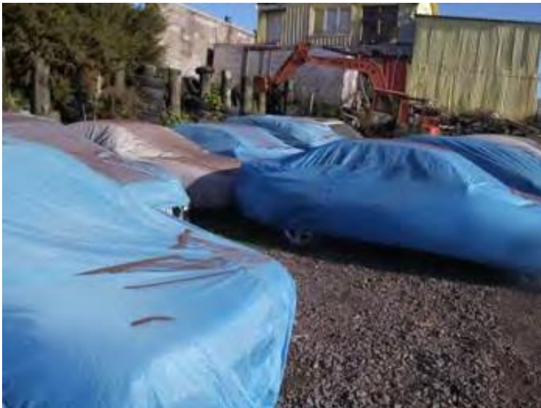
Figure 11 Tower painting in an industrial setting showing garnet debris falling onto covered cars.
