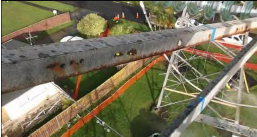
Figure 9 Tower corrosion
