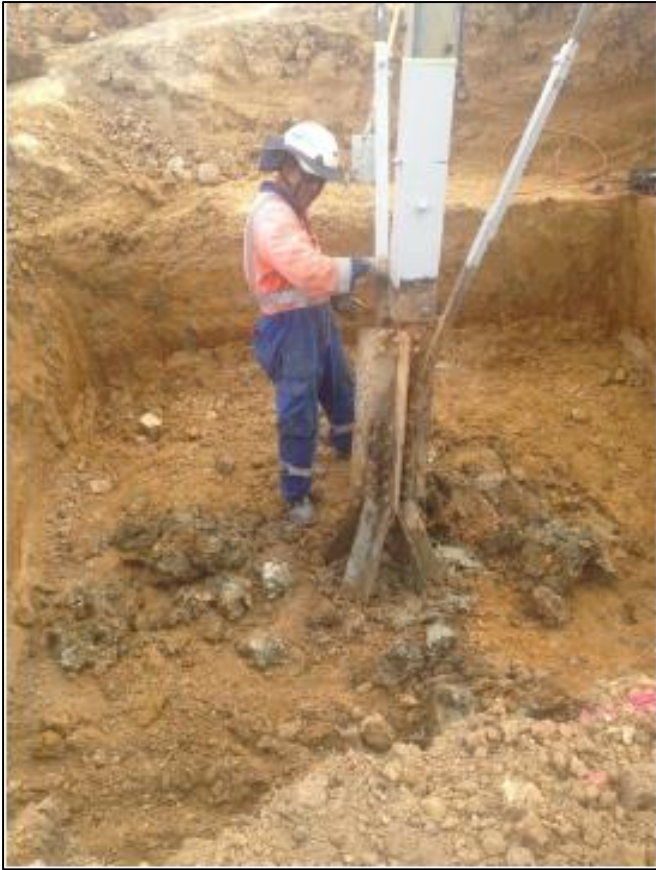
Figure 8 Land disturbance for grillage foundation strengthening.
