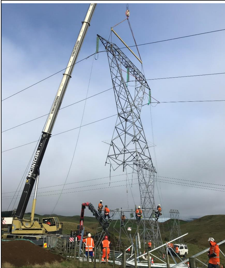
Figure 14 Parallel Body Extension being installed on the BPE-WRK-A line.
