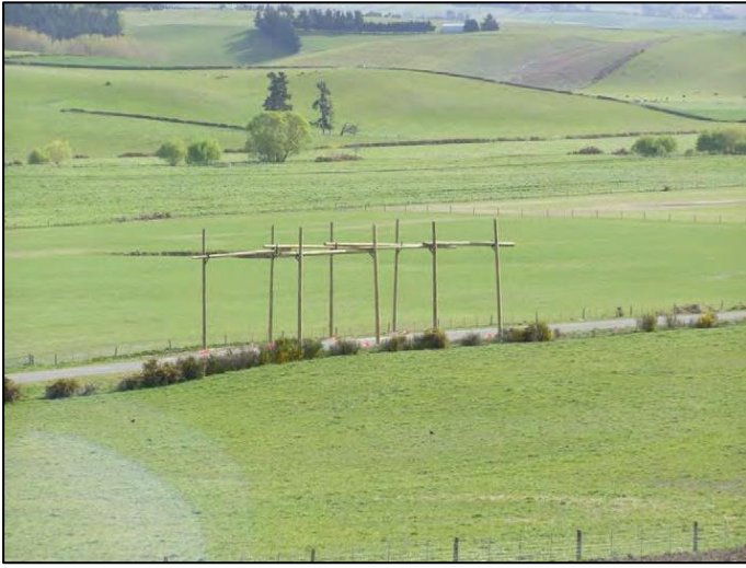
Figure 17: Typical hurdles installed to mitigate potential conductor drop during wiring.
