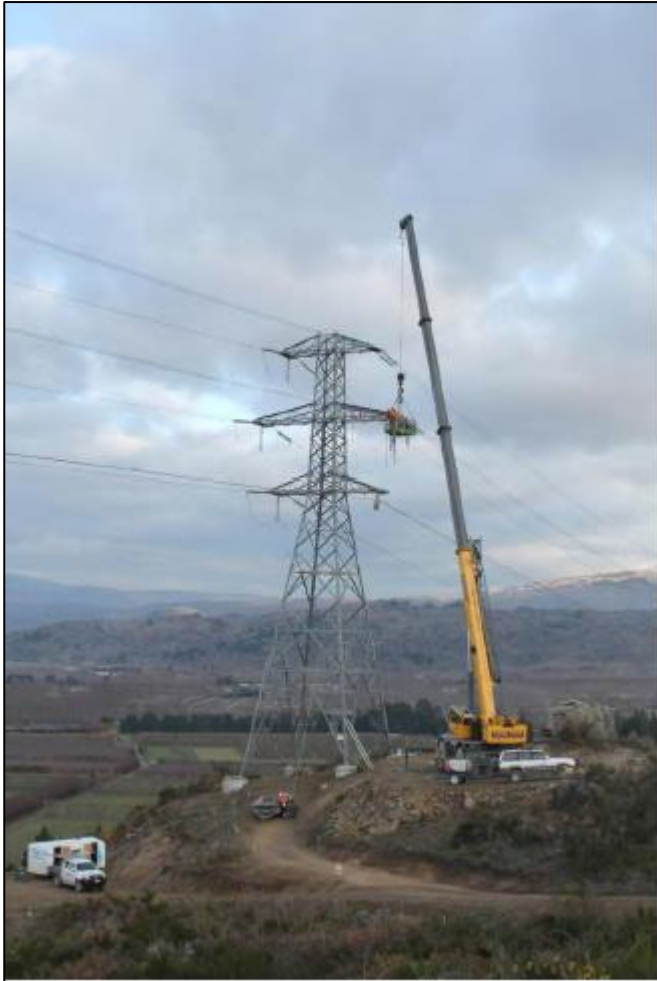
Figure 22 Example crane access required for cross arm and insulator works
