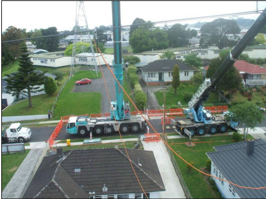
Figure 19: Reconductoring in an urban setting
