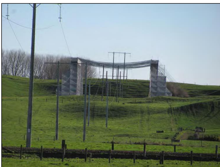
Figure 16: Scaffolding protection structure for stringing
