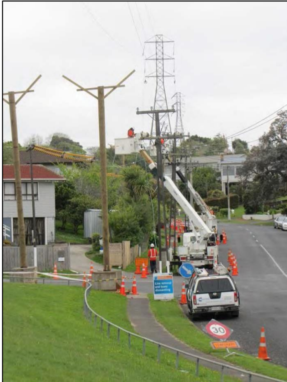
Figure 20: Removal of copper conductor
