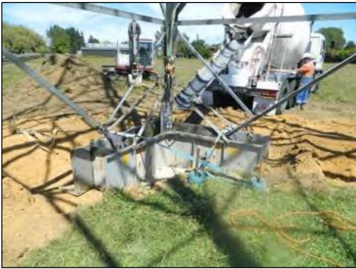
Figure 7 Tower Grillage foundation replacement
