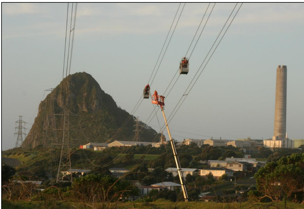
Figure 15: Conductor trolleys on duplex conductor
