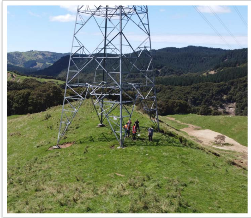
Figure 2. Earthworks at Transmission Gully
