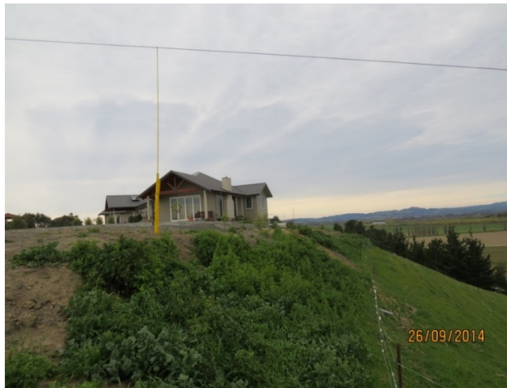
Figure 5. Hastings ground clearance violations
