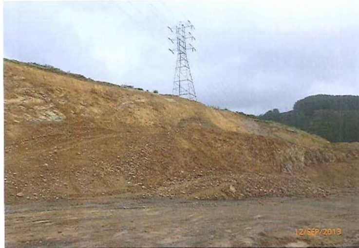
Figure 1. Earthworks in Porirua
