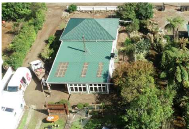
Figure 15. Debris flow deposition around a house in Granity. Approximate depth of inundation is <0.5m. Photo: BDC
