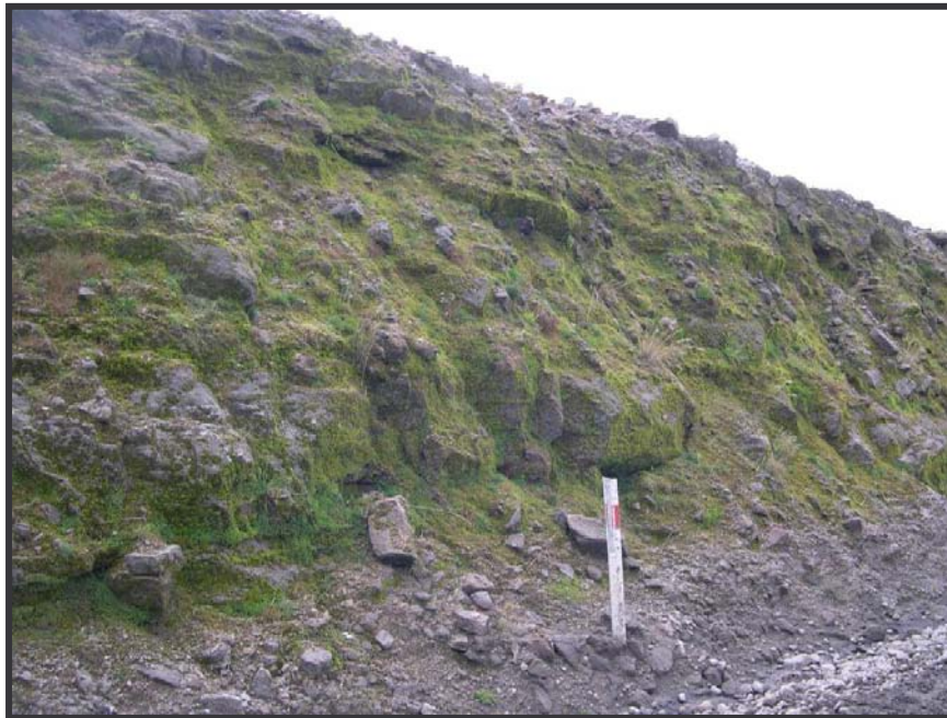
Figure16. Moss and other colonizing species hydroseeded (with some higher plant seeds) onto a rocky road cutting.
