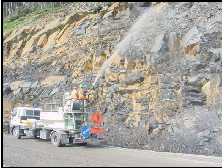
Figure15. Hydroseeding mosses and other colonizing species onto a roadside rock face.
