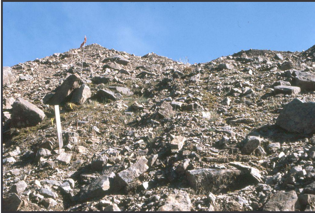
Figure 17. Bouldery angle-of-repose side-slope of an overburden waste rock dump, 2 years after hydroseeding with mosses and other colonizing plant fragments and native seeds.
