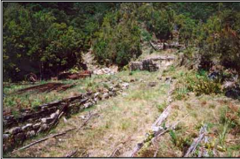
Figure 24 Cable guide wheels at the Middle Brake. These are situated in the central railbed where the loaded wagons were rolled to the lip of the lower incline. They guided the main hauling cable.
