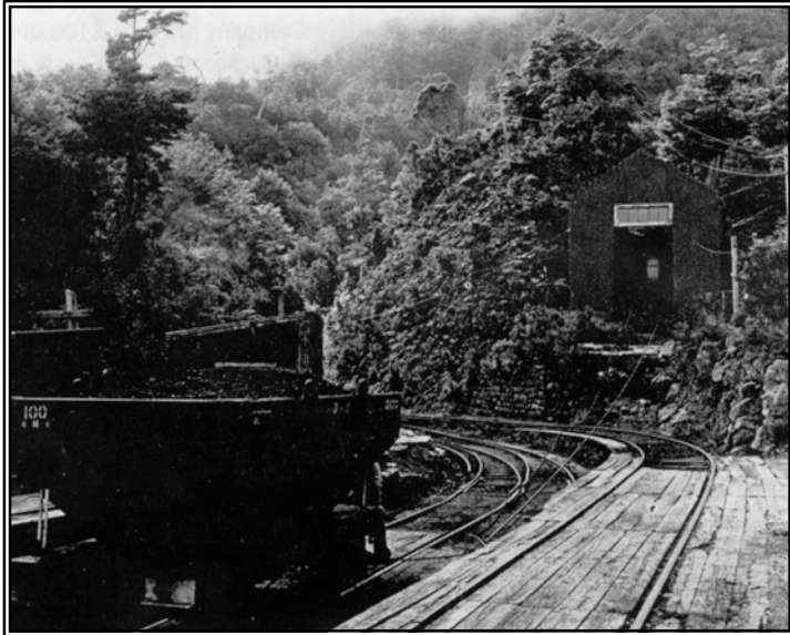
Figure 18 A 'Q' wagon and the brake shed at the Middle Brake, looking back towards the upper incline. (G.T. Radcliffe, with permission, N.Z. Railway & Locomotive Society).
