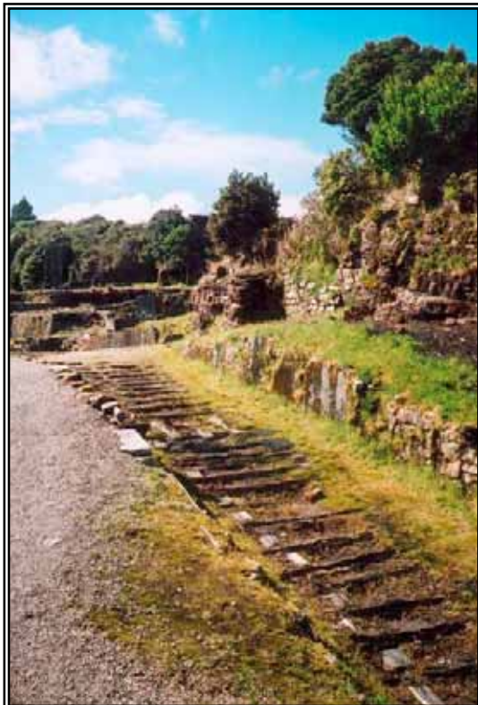
Figure 11 The top of the upper incline in 2006, before rail laying started. The original sleepers of the incline were still clearly visible.
