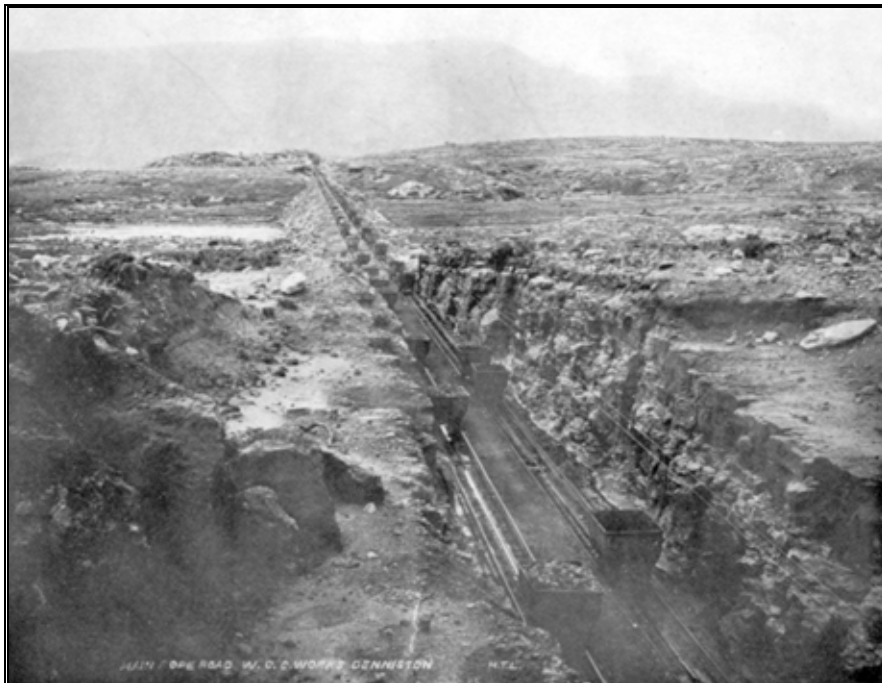
Figure 47 The rope road between Burnett's Face and the Brakehead in about 1906. (Morgan & Bartrum 1915)
