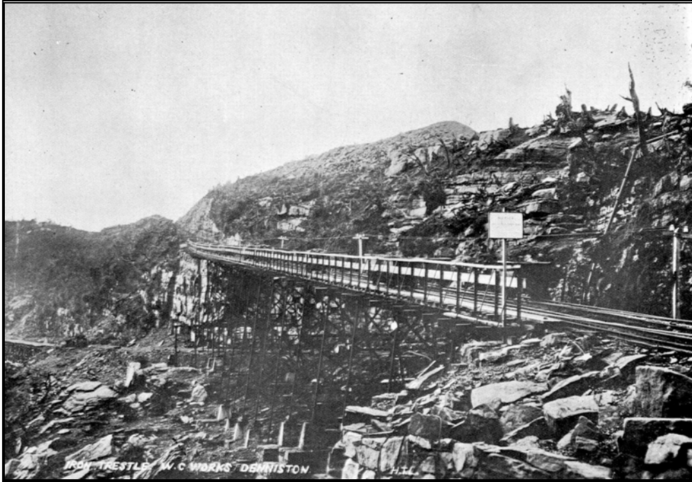
Figure 48 The rope road trestle just past the workshop site in about 1906. The old tramway to the Banbury Mine can be seen to the left, at a lower level than the far end of the new trestle. (Morgan & Bartrum 1915).
