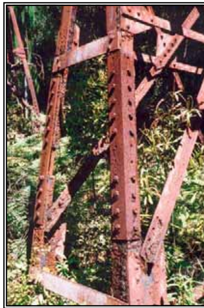
Figure 16 (right) A detail of the legs of one of the piers of Brown's/McDonald's bridge on the upper incline. As can be seen, some of the steel members are extremely rusty. It is not known whether the angle irons bolted to the legs were to raise the structure or to repair rust-weakened areas.
