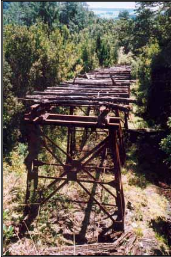
Figure 16 (right) A detail of the legs of one of the piers of Brown's/McDonald's bridge on the upper incline. As can be seen, some of the steel members are extremely rusty. It is not known whether the angle irons bolted to the legs were to raise the structure or to repair rust-weakened areas.
