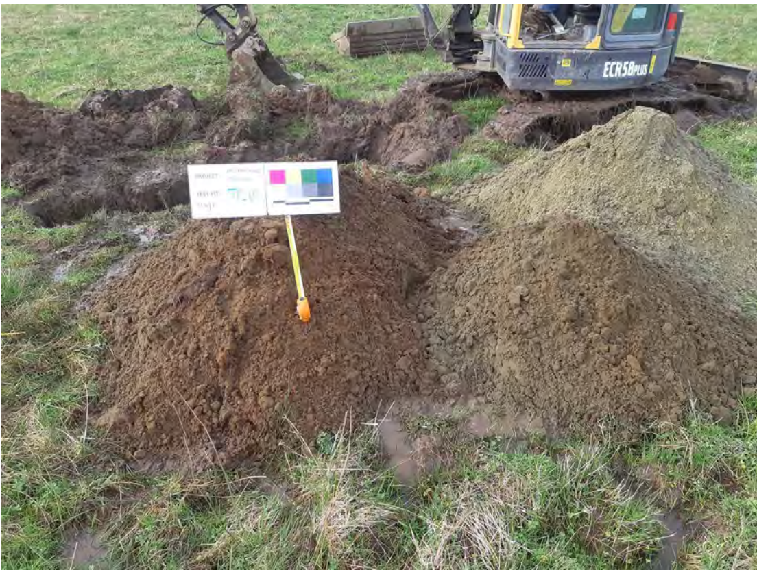
Spoil photo TP_02
