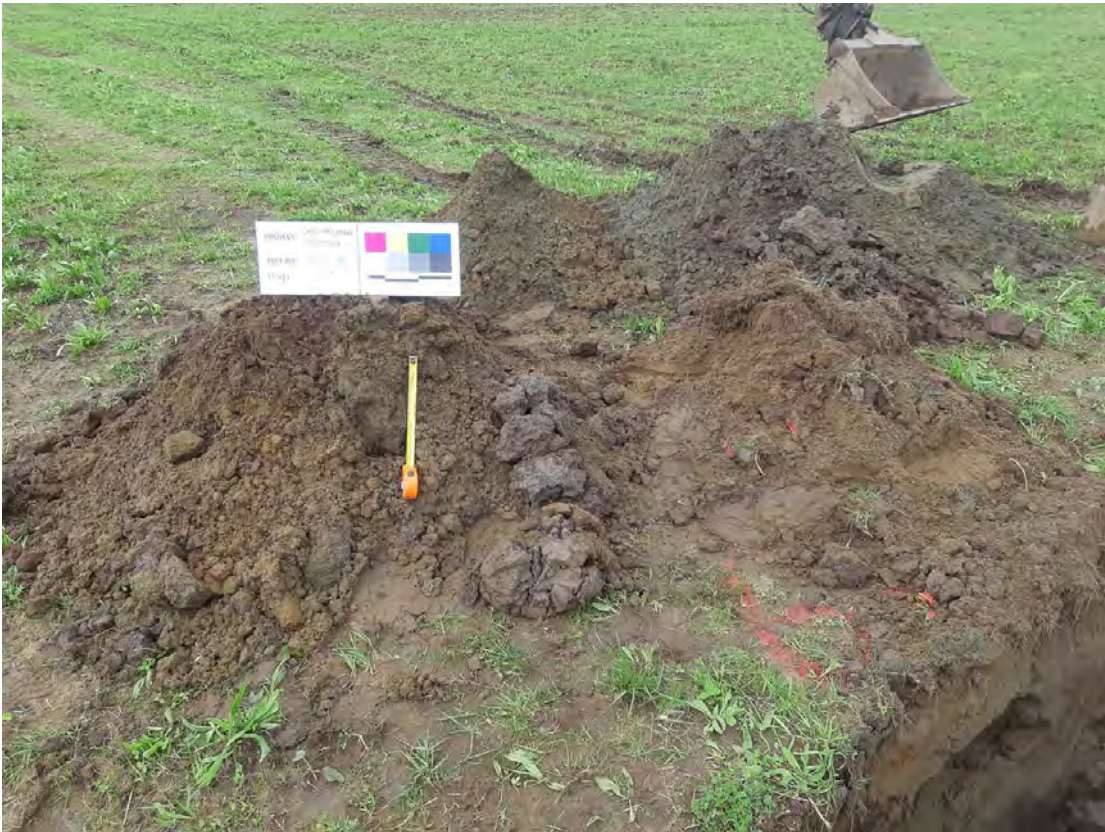
Spoil photo TP_09
