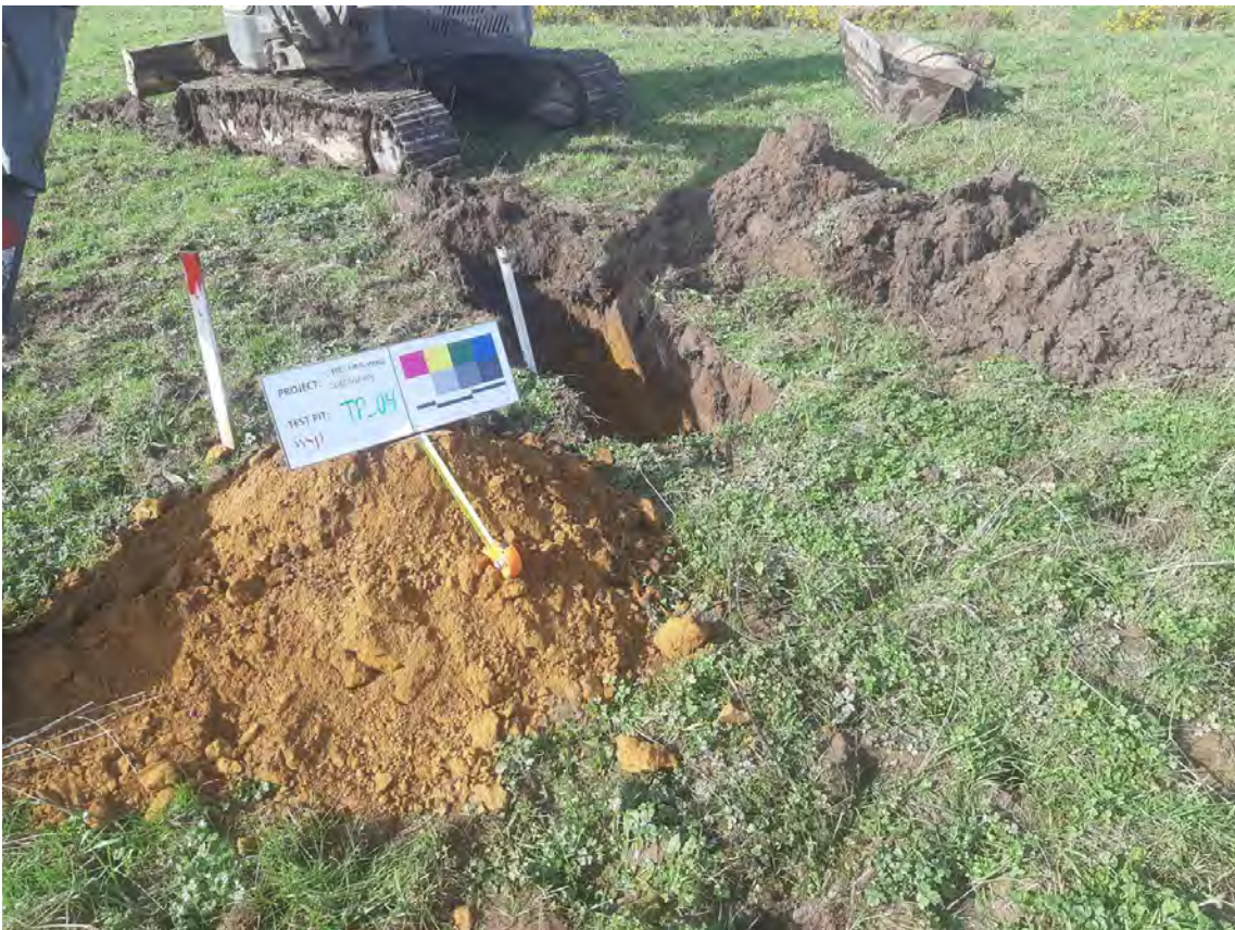
Spoil photo TP_04
