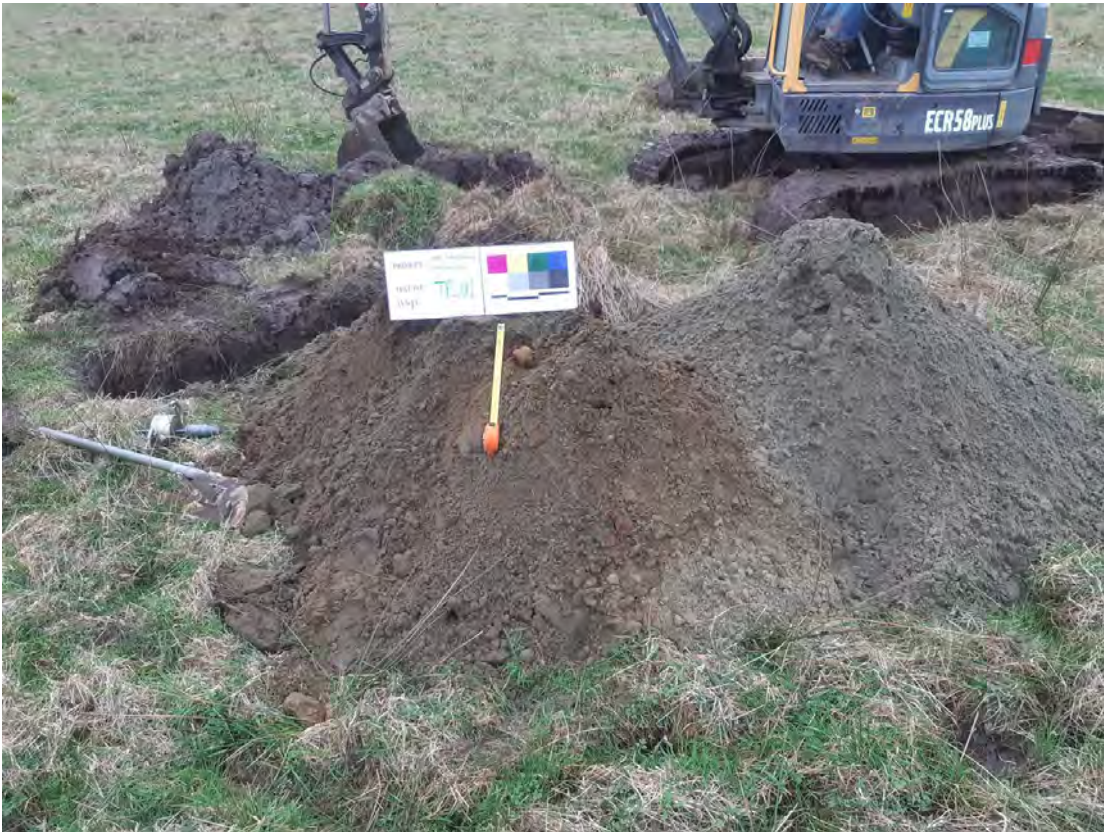
Spoil photo TP_01
