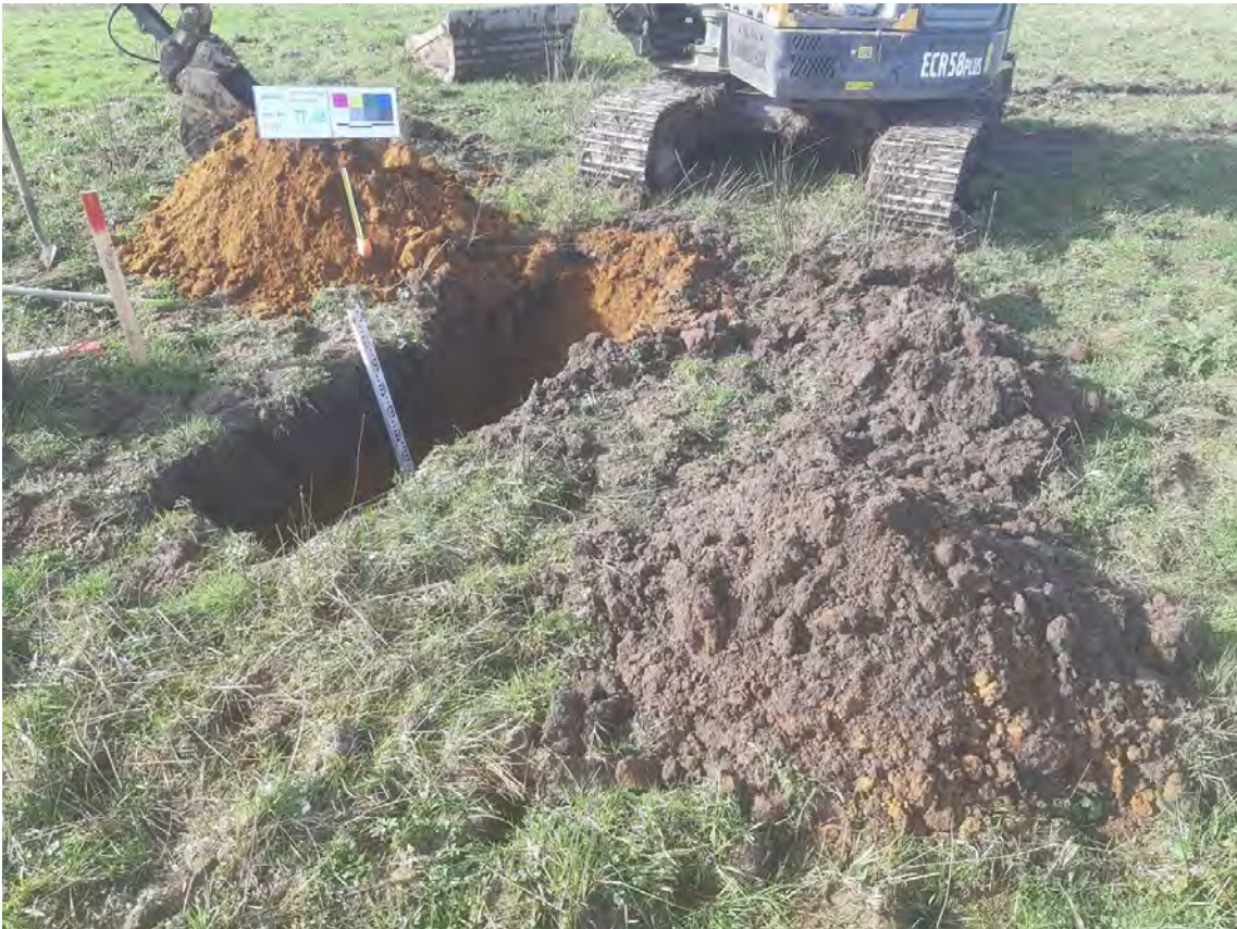
Spoil photo TP_03
